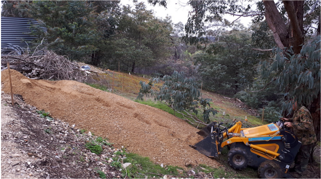
Compacting the soft road base to construct the access ramp.
